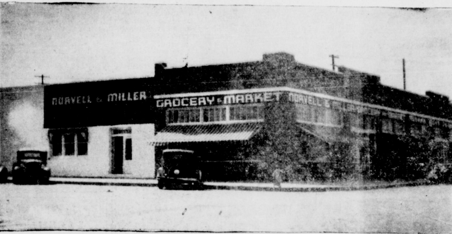
Front and side view of the big Norvell and Miller grocery store which is being formally opened this week at D Ave. and Tenth St.
