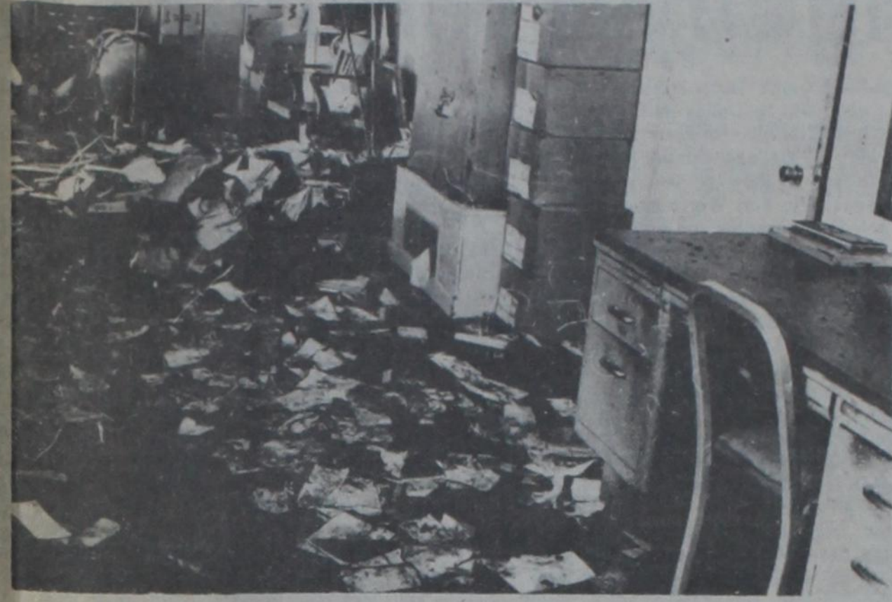
WHERE IT ALL STARTED ... The heating system [with vent at bottom] malfunctioned
