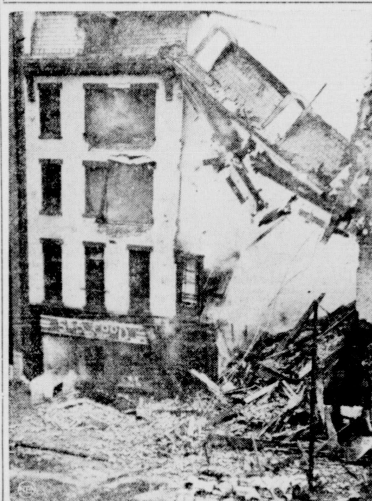
At the very moment the roof collapsed, the camera recorded this picture of the burning warehouse at Syracuse, N. Y., where eight firemen died when they were trapped beneath tons of debris.
