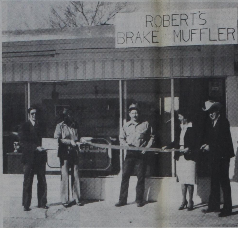
ANOTHER NEW BUSINESS—Robert's Brake and Muffler was officially opened as a new Dimmitt business last week when a ribbon was cut by the owner, Robert Daniel, assisted by Chamber of Commerce officials. From left
