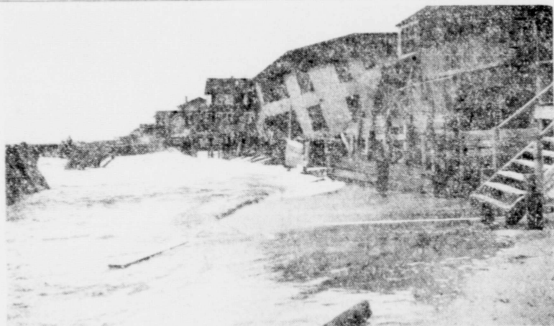
OCEAN AT THE DOOR—Ten blocks of two-family houses and summer bungalows turned into twisted wreckage by storm and gales, have been washed into Atlantic Ocean at Long Beach, New York. Crews of workers are now building emergency bulkheads to help houses still standing resist strong pull of swollen tides.
