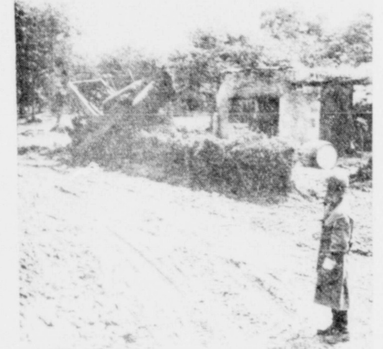
BULLDOZERS STOP AT NOTHING —Sweeping out underbrush in France, business ends up under a particularly heavy load. It's because it is wider than for Allied military traffic in Normandy.
