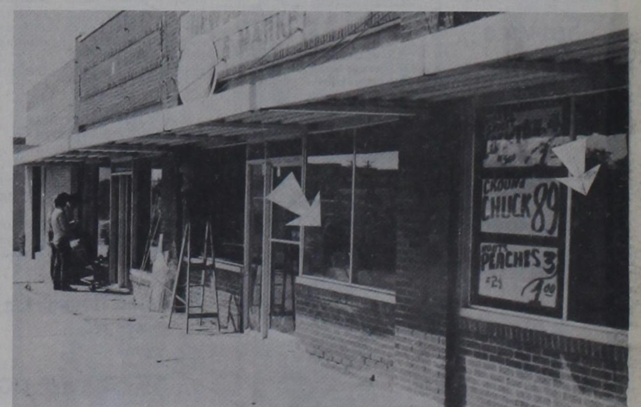
ARROWS SHOW broken windows in Hart buildings as workmen in the background start replacing glass Sunday morning. Victims were the post office, bank, Nora Lee's No. 2 clothing store and Pay & Save Super-
