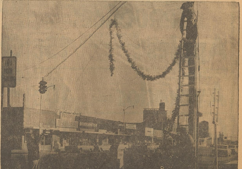
CHRISTMAS DECORATIONS were hung in downtown Dimmitt last week as preparations are underway for the celebration of the Yule season. Putting up the decorations are city employees Sam Maynard (at the bottom of ladder), Buck Raper (on ladder) and Amos Garcia. —Staff Photo
