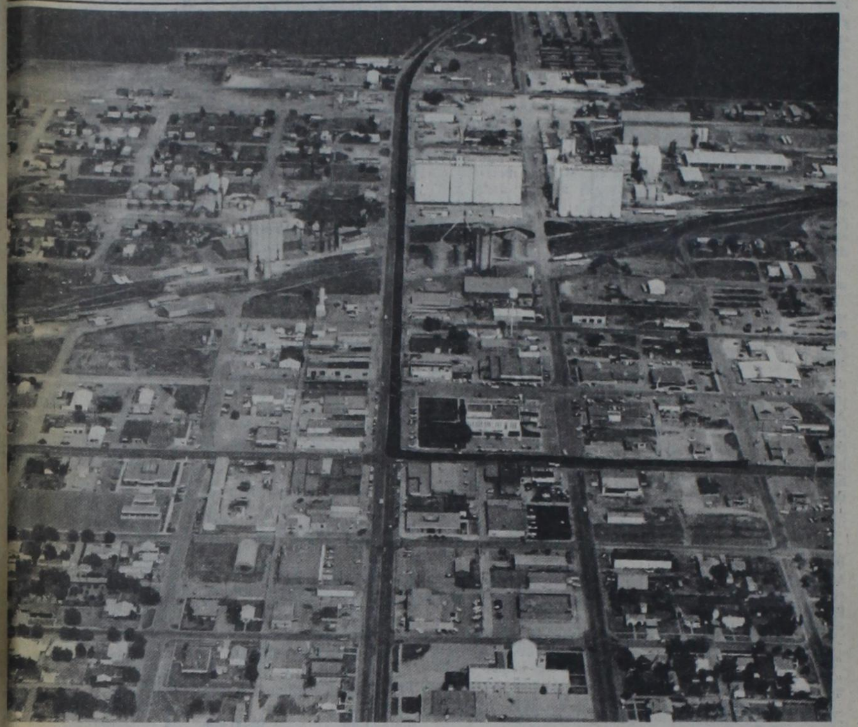
FIRST PHASE of the highway reconstruction project in Dimmitt will be the excavation of the south half of State 86 and the east half of US 385 as indicated by the blacked-out area. Workmen will begin Tuesday on East 86 (top), just beyond the Highway Dept. maintenance warehouse, and will tear out half of the highway to the Broadway-Bedford intersection, then will turn south and take out the east half of US 385 for two blocks.
