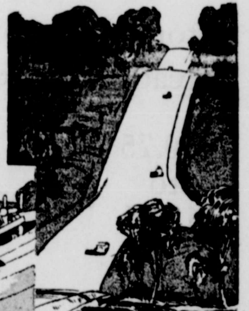
Very seldom are hills as steep as this. The average grade of highway hills is seven per cent. This hill is 25 per cent and a car must be good to make it.
