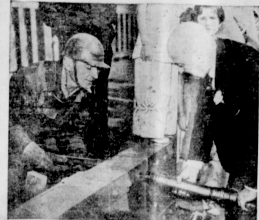
The last rivet was recently driven in the Golden Gate bridge at San Francisco. With many notables witnessing the ceremonies, a crew of iron-hatted riveters drove a golden rivet into the span, signaling completion of the structural steel work.
