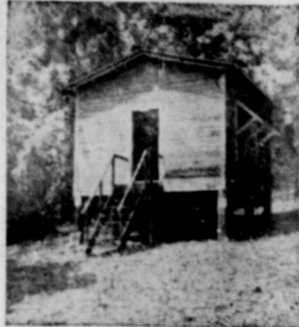
Panama test house. This photo shows that treated wood had not been attacked by termites.
