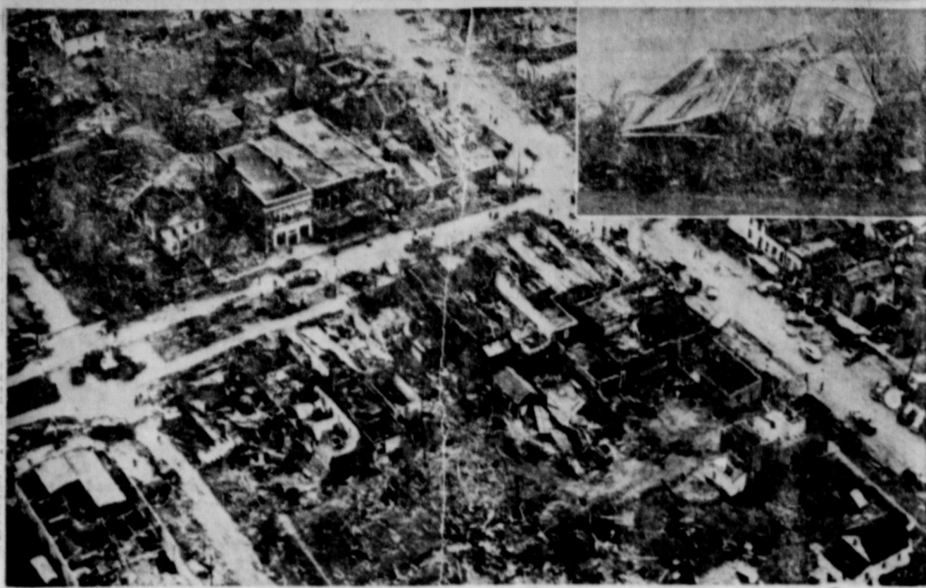
SHATTERED BUNKER HILL . . . The word "tornado" invariably calls to mind two accompanying descriptive terms, "death and destruction," and in the case of the twister that howled through west-central Illinois those adjectives were as appropriate as ever. It cut a furious swath through an area 50 miles wide and 100 miles long, leaving behind a death toll of 31 and a trail of shattered residences. Hardest hit community was Bunker Hill, almost completely destroyed by the force of the tornado. Inset shows a closeup of one of many houses that were shattered like cardboard toys.
