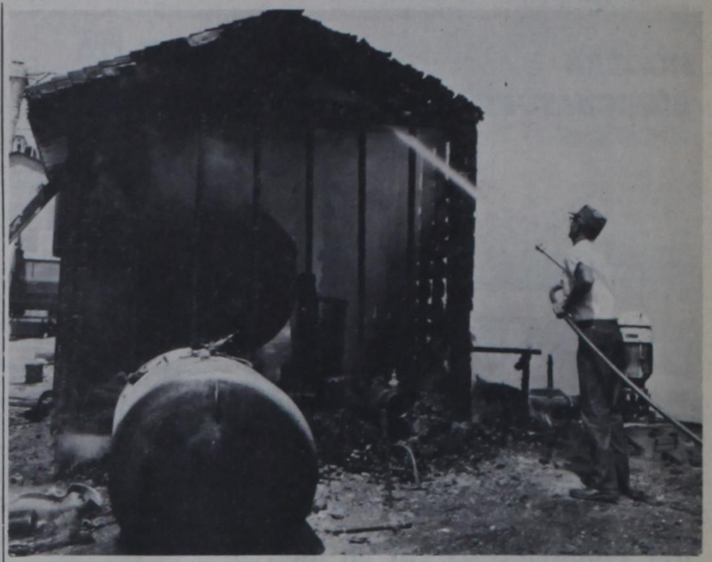
SATURDAY FIRE—This pump house at the Bud Hill farm and feed lots northwest of Dimmitt was destroyed by fire Saturday morning after butane from the tank in foreground accidentally ignited. Here, Fire Chief Harlan Dodd extinguishes flames around the ruined pressure pump inside the pump house. When the fire first started, Hill reported, the butane tank shot flames 50 to 100 feet through the air to the right, eventually igniting the pump house.
