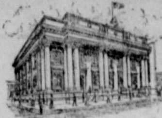
Main at Murphy Street
