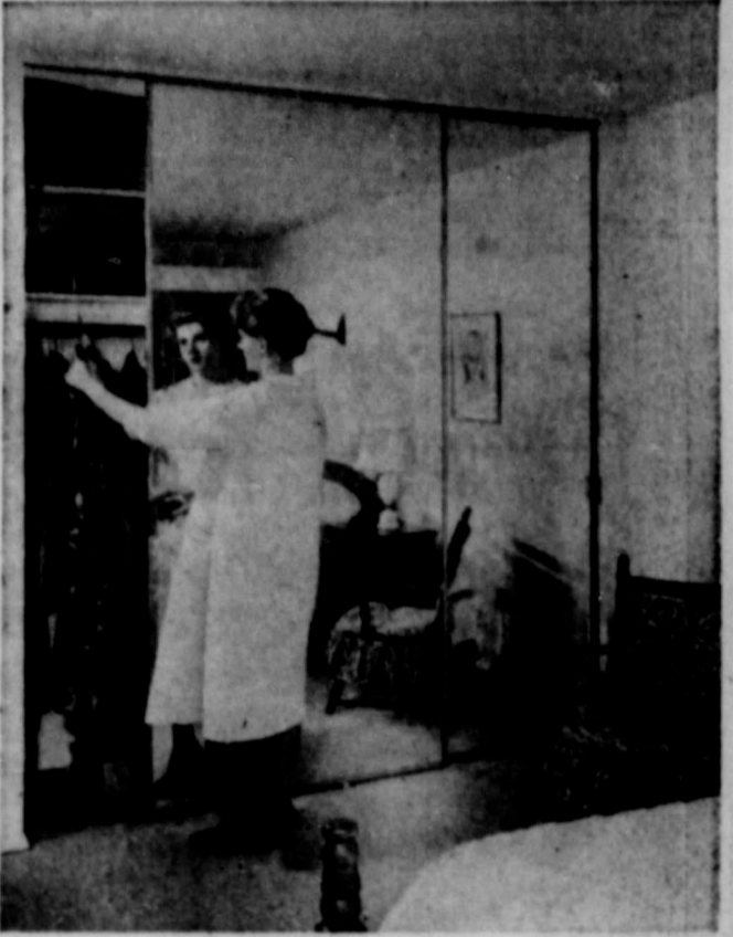
HERE'S AN IDEA on how to brighten a drab closet and make it more practical. This bedroom storage area is enclosed with sliding doors of Parallel-G-Plate mirror, which increase the light and add a feeling of spaciousness to the room. Ceiling-mounted tracks eliminate the solid bulkhead found above conventional closet doors, and allow the full-length mirrors to provide maximum storage and viewing area.
