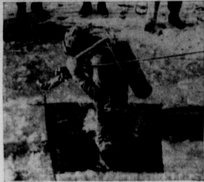
CHILLY DIP —Man with a cool job, diver Al Herman, drops through a hole in the ice of Wirth Lake, Minneapolis, Minn., to inspect dock piling.
