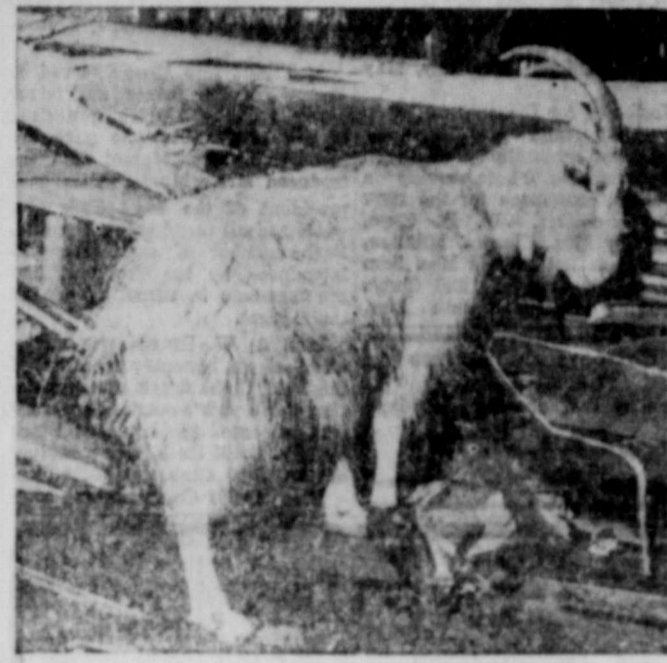
WHERE THE BARN WAS—A homeless goat wanders amid rubble left by a lightning bolt swept through Wilburton, Okla.
