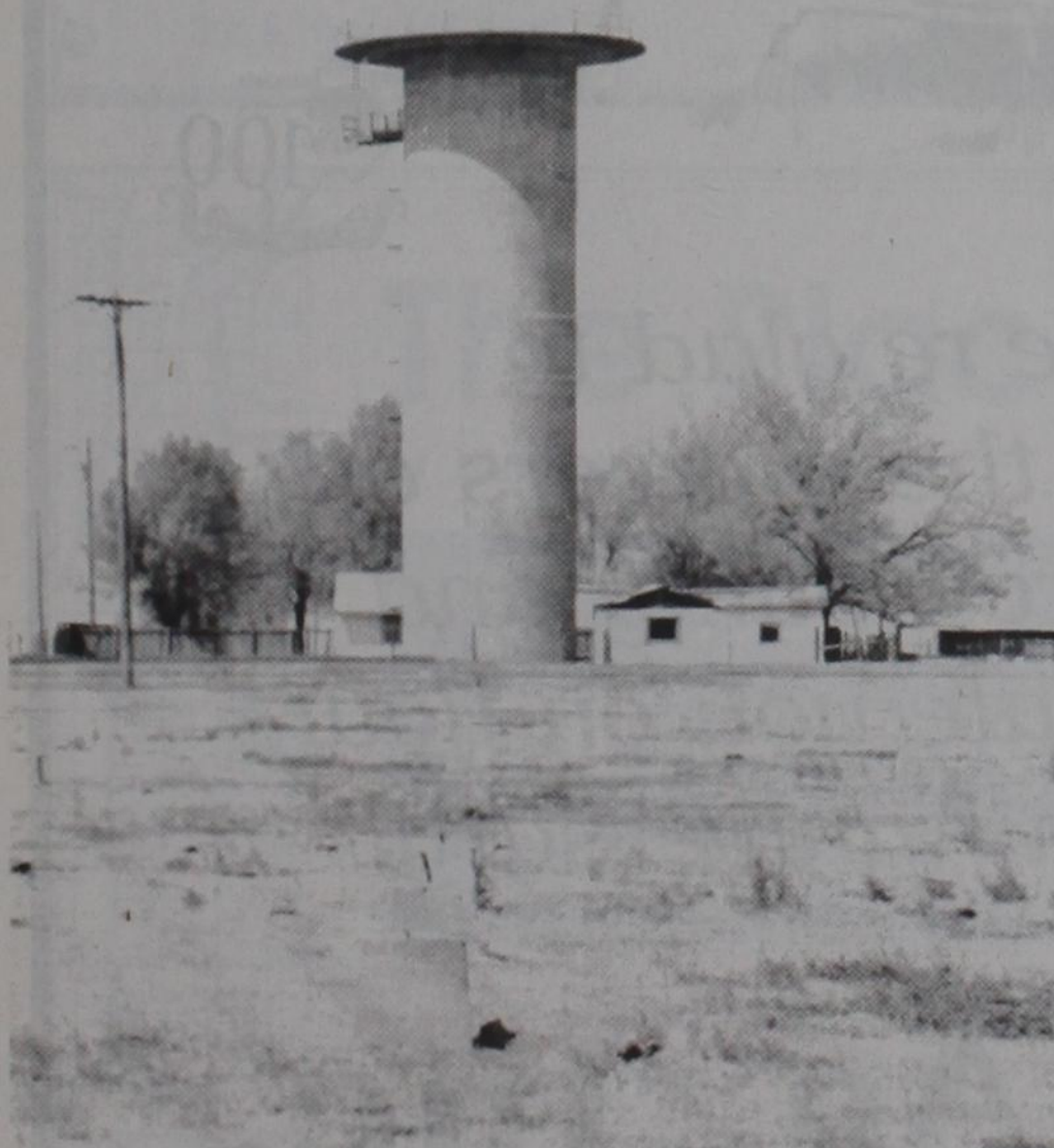
THE WATER TOWER'S concrete cylinder, minus its tank, stands as a lone sentinel over the other remnants of the Hereford POW Camp. The tower's wooden ladder is still intact, although the screening for the ladder's safety tunnel is gone. The tower is now unsafe to climb. Rising out of the native grass in foreground are the concrete piers, sunk four feet into the ground, which supported many of the camp's buildings.
