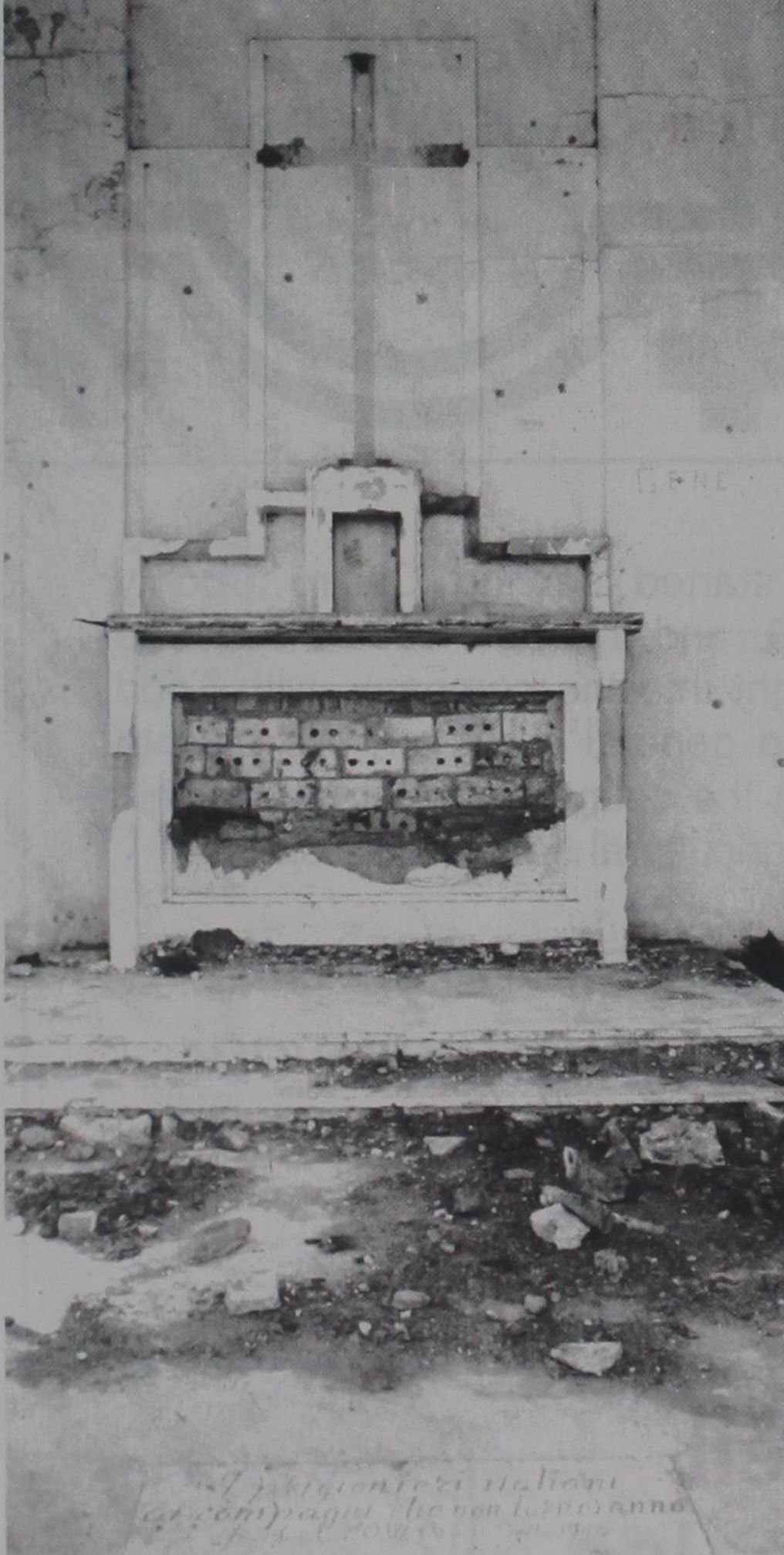
INSIDE THE CHAPEL, despite years of vandalism, one can see the meticulous craftsmanship that went into the construction of the memorial. The Italian prisoners worked their plaster for the walls and altar until it approached the smoothness of granite and marble. (Photo by Don Nelson)
