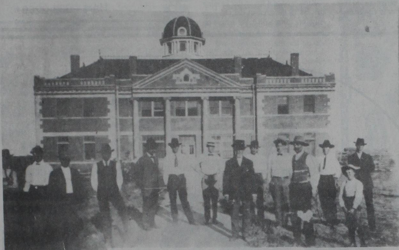
EARLY-DAY COMMISSIONERS POSE AT SECOND COURTHOUSE ...Built in 1906, torn down in 1930 to make way for the present one
