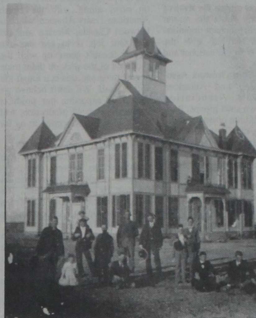
CASTRO COUNTY'S FIRST COURTHOUSE
