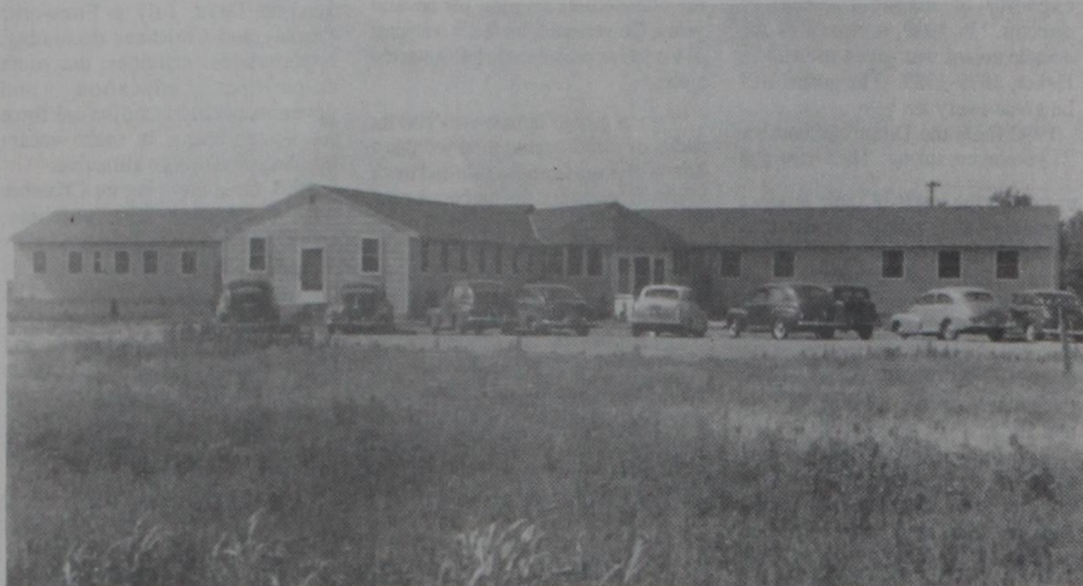
HOSPITAL BARRACKS —This building housed the first Plains Memorial Hospital in 1964. It was made from the old hospital barracks building which was at the Hereford Prisoner of War Camp in Castro County. File Photo
