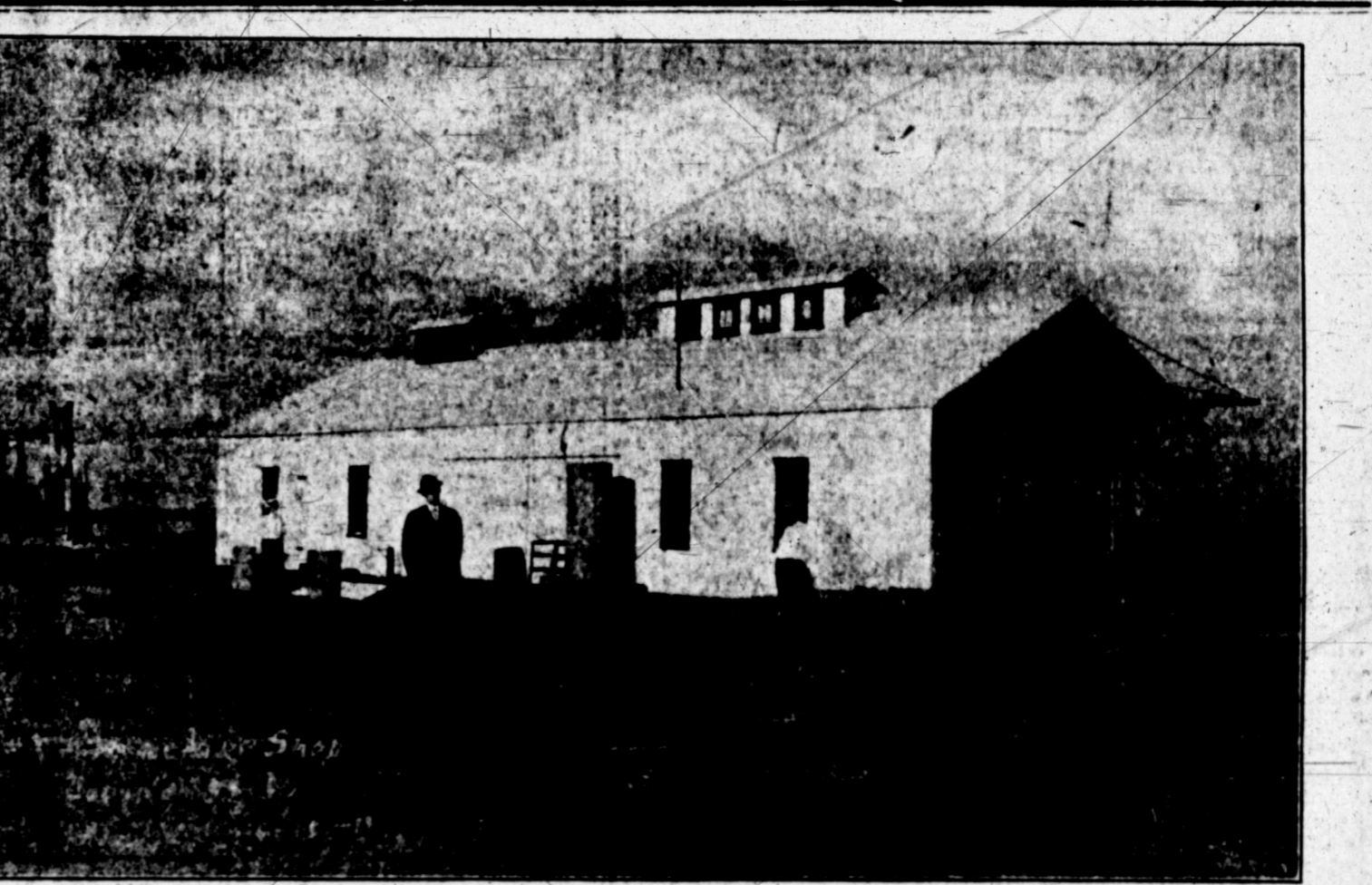
Machine Shop at Electra.
