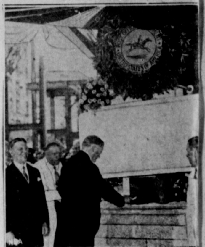
Using the same trowel which President Washington once used in similar ceremony, President Hoover laid the cornerstone of the new U. S. Postoffice Department building, on which the government going to spend $10,500,000. That's Postmaster-General Walter Brown at left.
