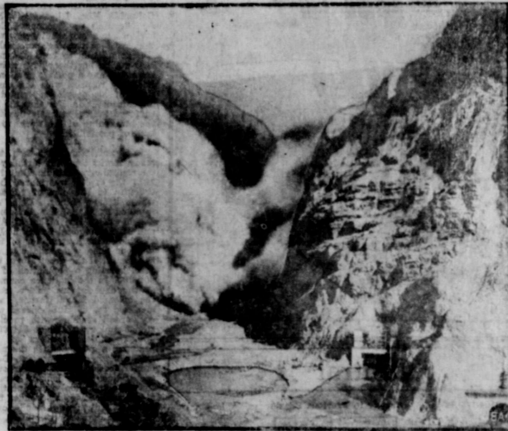
With a deafening roar, this titanic blast of dynamite ripped the sides of Boulder Canyon, in Colorado, clearing the way for the gigantic Hoover Dam which is to block the canyon and harness the horsepower of the Colorado river. Note the openings of three of the four diversion tunnels which have been drilled through solid rock from a point above the dam to a point below, to carry the waters of the river while the dam is being built in the dried river bed.
