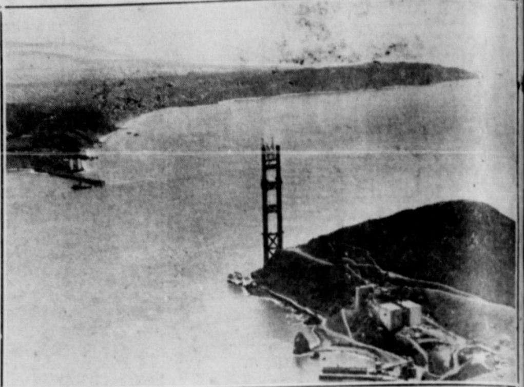
Like a mighty sentinel standing at the Golden Gate, the 740-foot tower in the foreground appears in the striking air view. Rising from Lime Point, it is the Marin county support for the cables and the 1,900,000-bridge that will span Golden Gate, famed entrance of San Francisco harbor.
