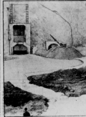
water poured down the spillway from No. 1 diversion tunnel to begin joyed such a record flow of tourtoo, lent Fish considerable money filling the mammoth reservoir of \$49,000,000 Boulder dam. In this picture the gigantic bulkhead gate of No. 4 tunnel was being closed Sewell. The hotels, railroads and at the rate of nine inches a minute to divert the water to No. 1 tunnel, where control gates direct the flow.
