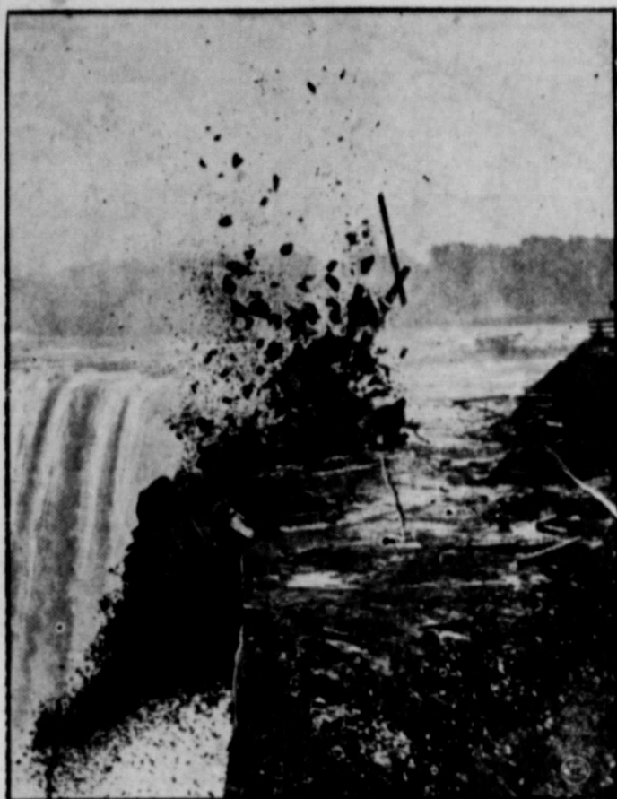
Niagara's roar was momentarily challenged as this man-made blast tore a 600-ton slice off Table Rock at the Canadian tip of Horseshoe Falls and sent it crashing into the gorge below. Fifty thousand holiday visitors watched spellbound as a second blast reduced the ledge, often called "Honeymoon Point," to half its former size. The dynamiting was undertaken to guard against possible rock slides from a crack extending 200 feet along the table.
