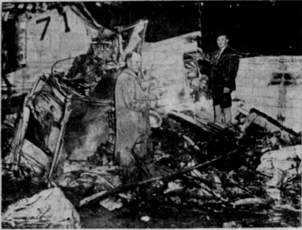
This is all that remains of the once-proud army bomber which crashed near La Grange, Ga., during a storm. Seven army men were killed and an eighth seriously injured.
