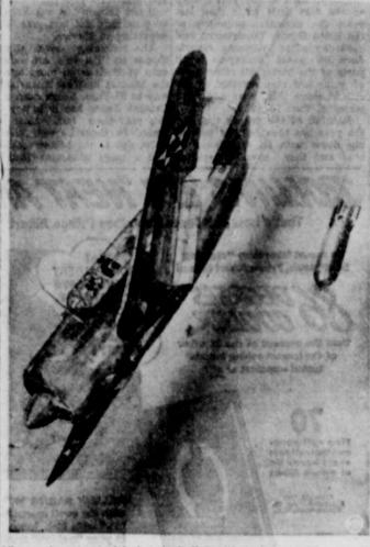
Like a gigantic steel-jacketed bullet with wings is this new dive Guiana, Jamaica, Trinidad and bomber, being readied for U.S. Navy trials at the Curtis-Wright plant, Buffalo, N. Y. The artist's conception shows it at the bottom of the dive, just after releasing bomb. Designed for aircraft carriers, the low-wing, all metal Curtiss XSB2C-1 has unusually heavy fire ower and carries increased bomb loads over long distances. It has
