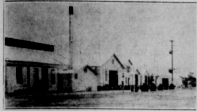
Above is shown the Eureka Tool Company's Ranger plant, one of the largest exclusive oil country machine shops in the Southwest. Work in the plant is done only by the best men obtainable and only the best steel and iron is used in work turned out by the $100,000 shop.
