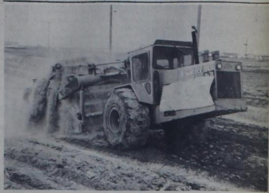
loader emerges from a deepening pit at Dimmitt Wheat Growers, Inc., with a load of dirt to fill the stem wall of the starch warehouse, first building in the coop's huge corn mill complex. Wet weather slowed the earth-moving operations Thursday and Friday, but now the bottom loaders are scooping at full steam.
