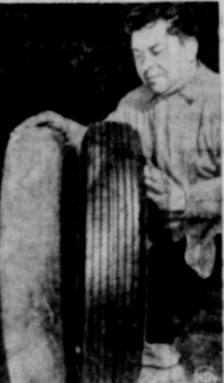
Here's the change that comes over an old tire during a retreading treatment. A New York tire shop attendant exhibits before-and-after samples.
