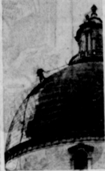
Dull gray war paint cloaks brilliance of $11,000 worth of gold leaf on dome of Massachusetts state house in Boston so it won't be a shining air raid target.
