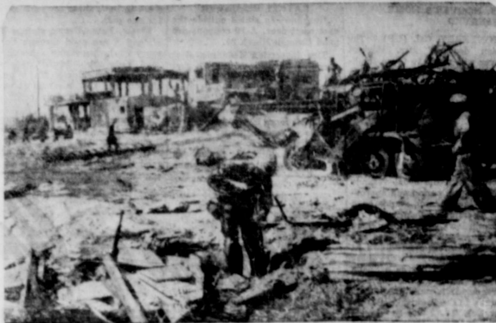
UNITED STATES MARINES are shown above digging foxholes on Namur island in the Marshalls. The burned out Nipponese mechanized equipment and the ruins of the big blockhouse, seen in background, show effectiveness of the American bombardment by sea, air and land (International Soundphoto)
