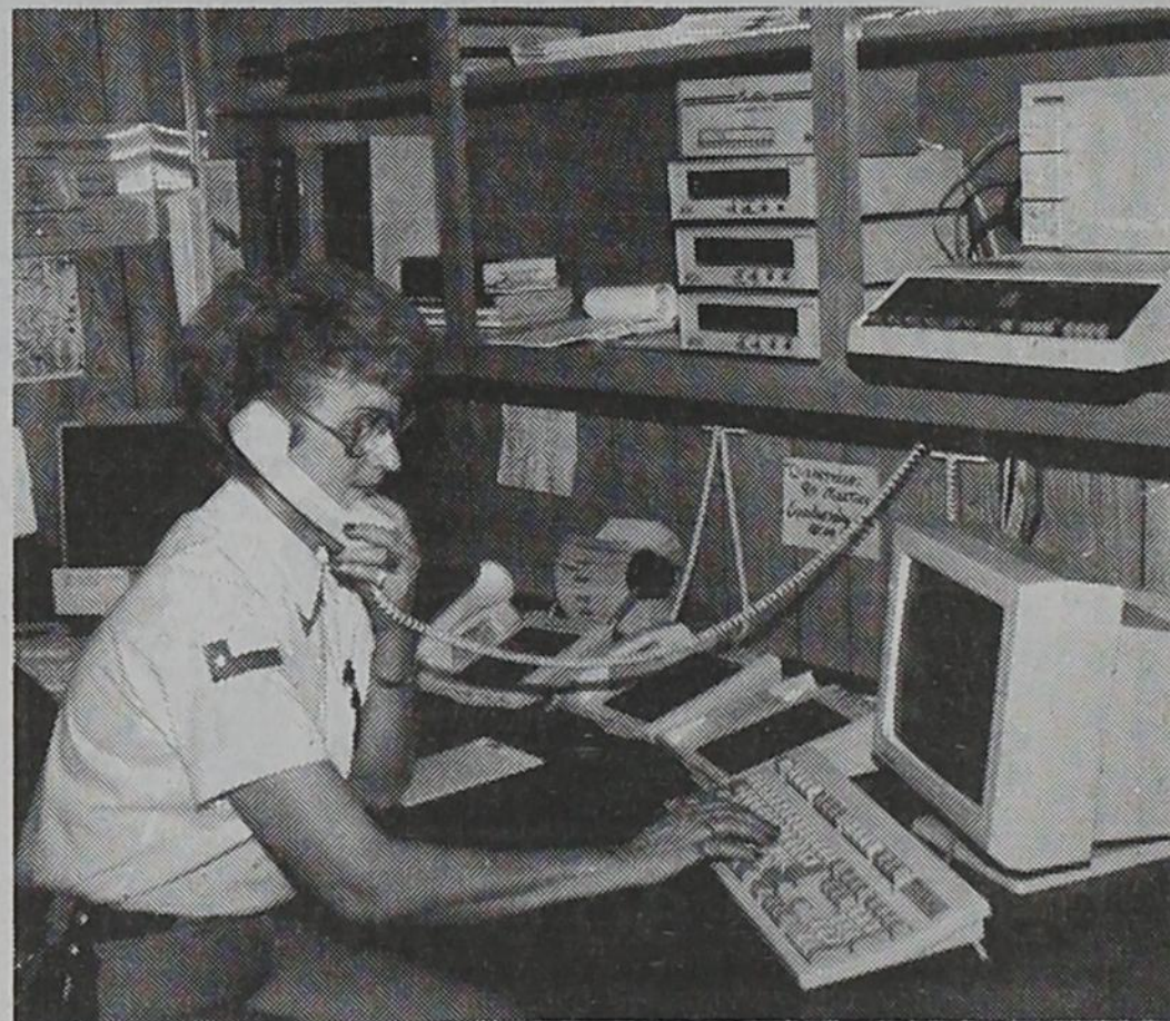
READY TO HELP — Castro County Sheriff's Dept. dispatcher Earlene West types in a telephone number on the 9-1-1 emergency communications system computer in the courthouse to see if the number is registered in the 9-1-1 data bank. Registered numbers will make emergency response times shorter. Photo by Deana McLain
