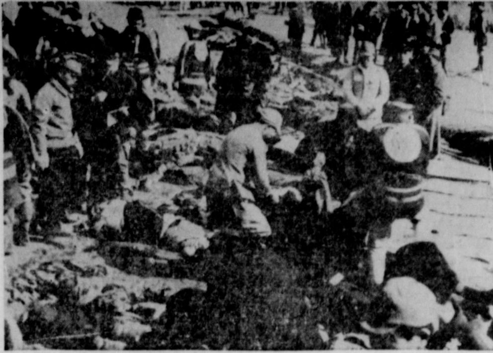
Costumed rescue workers, survivors and trainmen go about the grim task of identifying and placing the bodies of victims in a row on games mats after one of the worst railway disasters in the history of Japan. The last six coaches of an express train left the tracks on a sharp curve near the village of Hachioji, February 25, hurtling down a 30-foot embankment, killing 163 Japanese and injuring 249. No Americans were aboard. (NEA Telephoto).
