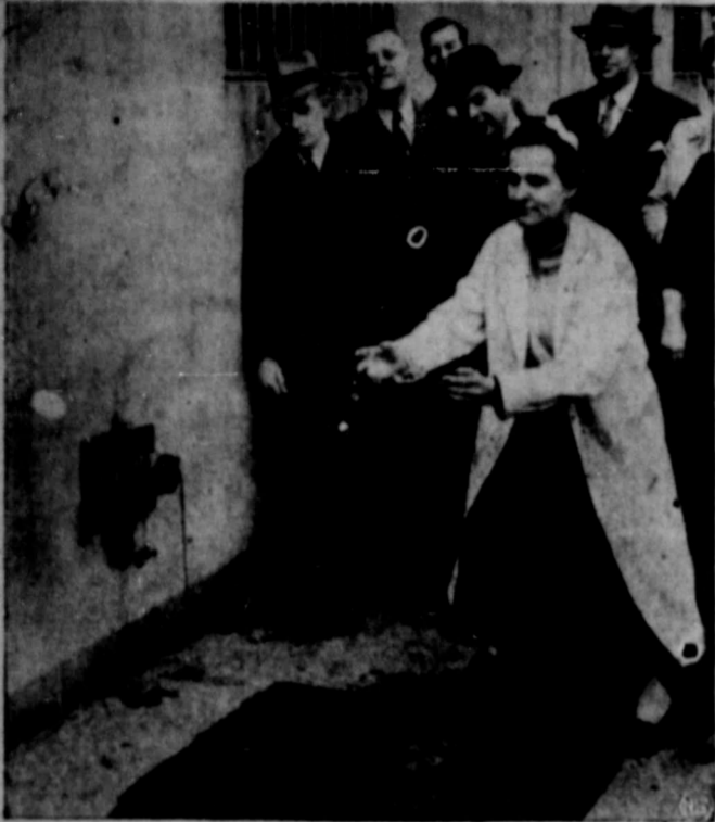
Fresh eggs, dropped from the roof of a 100-foot high building in New York City, landed without breaking and in fact bounced back as high as 35 feet in the air. Eggs landed on pad of sponge-like rubber containing millions of tiny, shock-absorbing air cells. Stunt was a demonstration by the New York Hospital-Cornell Medical Center and the U. S. Rubber Company in joint research on prevention of injuries in airplane crashes. Above, Margaret Agburn, research assistant, just misses catching bouncing egg seen at left.
