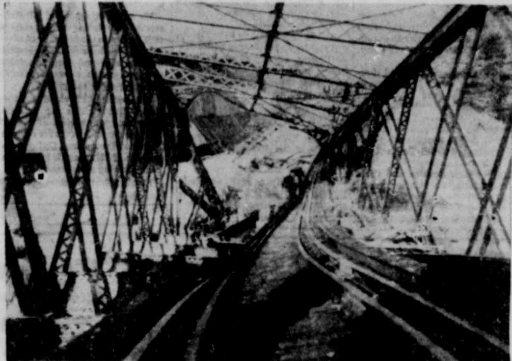
Twisted rails over this washed out bridge are a result of heavy rains which caused flood waters to burst through a dam in Rutland, Vermont. Ten families are believed to have perished in the roaring waters. (NEA Telephoto).
