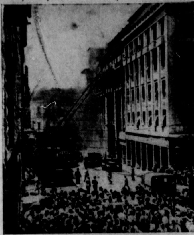
When the Soldiers' Pension Building caught fire in Athens, the blaze consumed virtually all Greek aid and UNRRA records. The headquarters of both UNRRA and the Greek-Aid Mission were in the structure. Conflicting reports on casualties list anywhere from three to 11 killed in the blaze which, the government says, was set by Communists.
