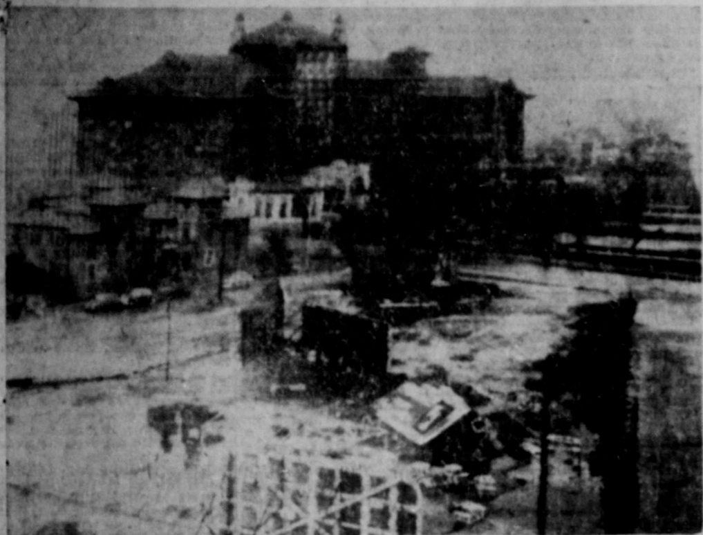
Wreckage of a watermelon parlor which was demolished when a 69 mile per hour wind struck Galveston is shown in the foreground. The famed Galvez Hotel, in the background, was undamaged. (NEA Telephoto).
