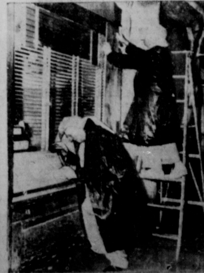
Carl Bachmann, left, and Ludwig Schmidt are boarding up a store front in West Palm Beach, Florida, in preparation for the hurricane which was expected at any time. Winds of 50 to 60 miles an hour were lashing the West Palm Beach seawall in advance of the center of the storm, which struck Wednesday. (NEA Telephoto).
