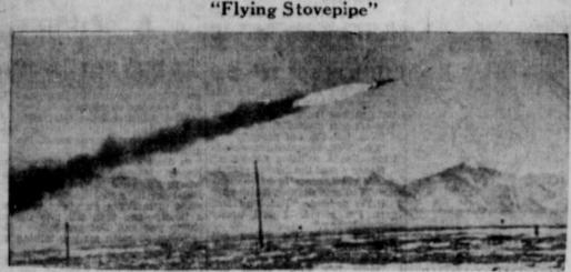
A "flying stovepipe" of the type which has attained speeds of 1500 mph, according to announcements made by the National Advi sory Committee on Aeronautics, streaks from its launching platform. In recent tests the missles have been launched from B-29s and permitted to drop into the sea off the testing area on the Virginia Capes. (NEA
