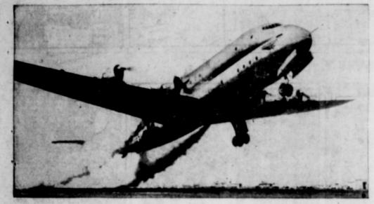
The Navy's 180-passenger "Constitution" takes off from a New York airport with the aid of six rockets. Engineers say that jet as sist permits the plane to shorten take-off runs nearly 24 per cent. Lockheed and Nav y pilots have been testing the "Constitution" preliminary to final acceptance by the Navy Department. - (NEA Telephoto)
