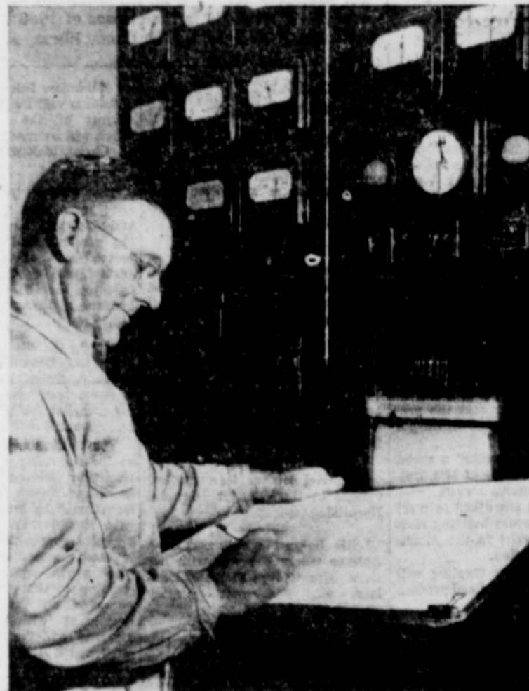
1. Close control of every process has enabled Baytown refinery to make its substantial contribution to your need for petroleum products. This is the control panel in one of Baytown's two catalytic cracking units, called "cat crackers." They enable Baytown to get more finished petroleum products from crude oil processed at the refinery.
