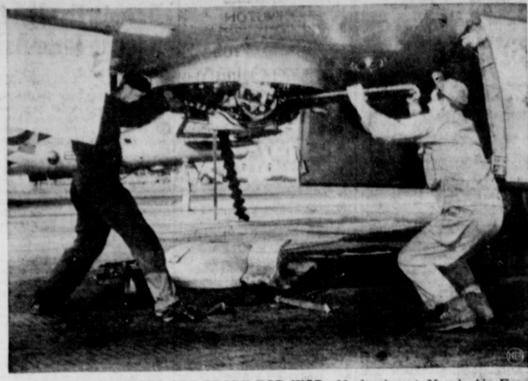
MARCH FIELD BOMBERS GET READY FOR WAR —Mechanics at March Air Force Base, Calif., install 50-caliber machine guns in bottom turret of a B-29 bomber which is being outfitted for combat duty. Three squadrons of B-29's from this base are awaiting final orders before taking off for Korea. (NEA Telephoto).
