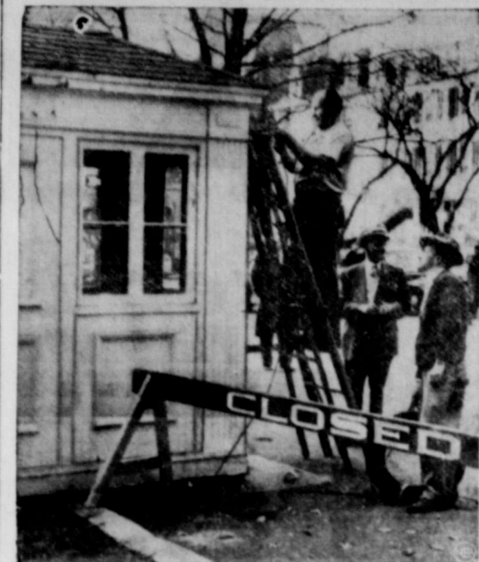
MORE PRECAUTIONS — As part of the program to provide greater protection for the President, a new sentry booth was set up across from Blair House. The street running alongside the White House (opposite Blair House) is closed and no one may enter unless a White House pass is shown.
