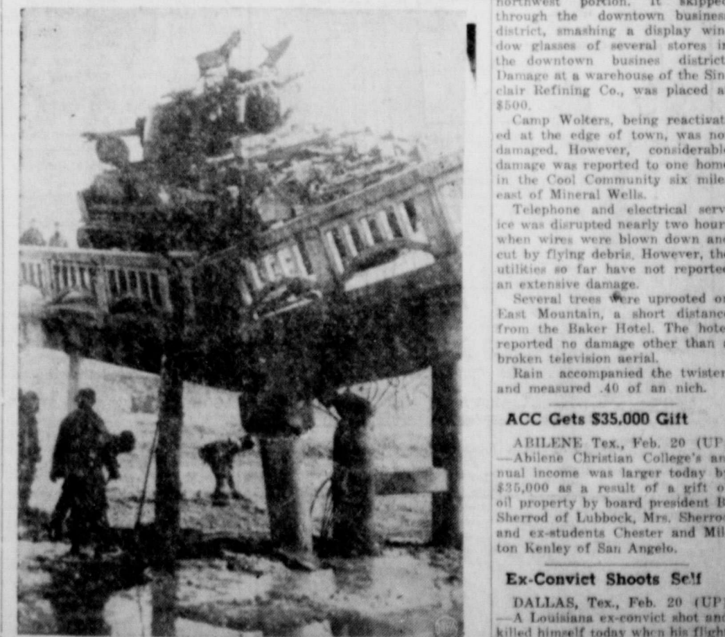
JOB FOR RETRIEVER—Men of the 8th Engineers Battalion, 1st Cavalry Division put logs under weakened support of bridge near Yangzi, Korea, to prevent its collapse. The new strength will support the bridge until a tank retriever can remove the M-4 which is stranded. (NEA Telephoto).
