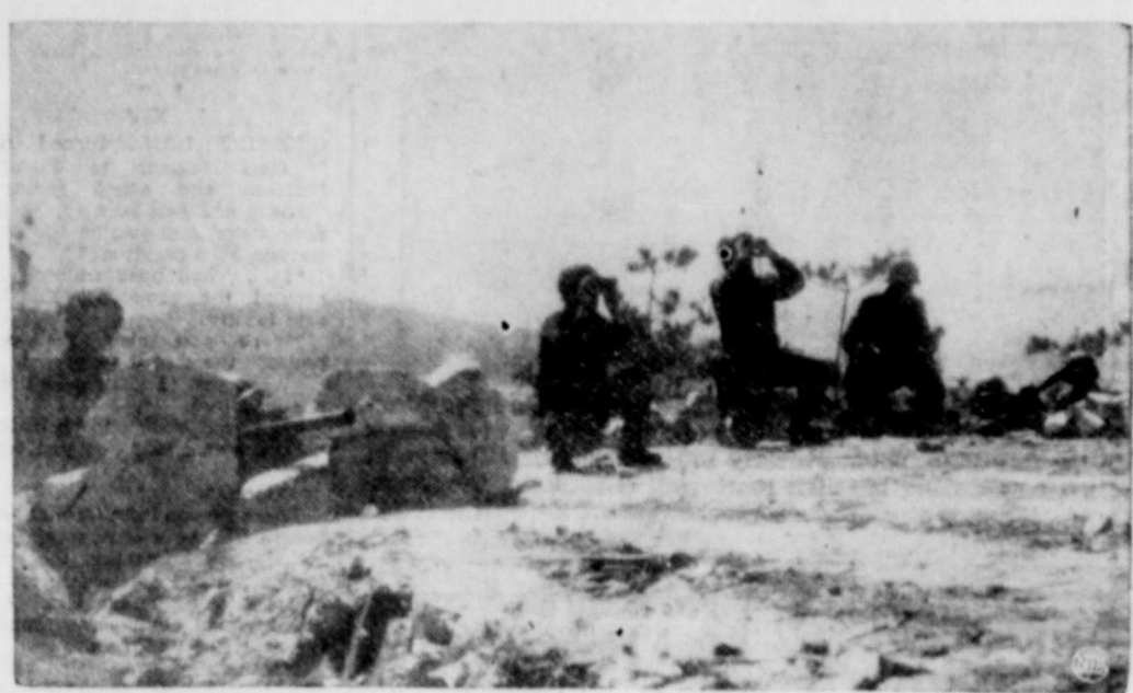
UN ROAD BLOCK—Using boulders for a barricade, a UN force throws up a roadblock in North Korea in case of any movement by Red forces north of the 38th parallel. (NEA Telephoto).
