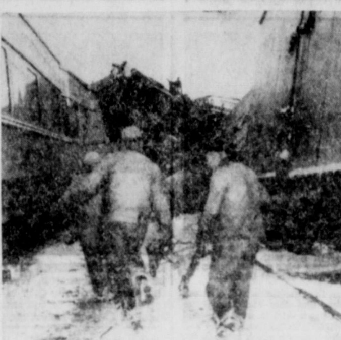
WRECKAGE TAKES ITS TOLL—Rescuers carry a body between the City of Los Angeles and the freight train in which it was thrown against the City of San Francisco rammed her, killing at least 20 and injuring scores. (NEA Telephoto).
