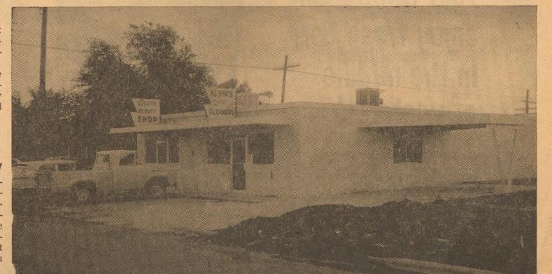
NEW BEAUTY SHOP AND DRY CLEANERS BUILDING owned by Mr. and Mrs. Alvin Frazier was erected by Killingsworth Construction Company of Dimmitt. Featured in the 36'x80' building are professional dry cleaning facilities, coin operated machinery for do-it-yourself cleaning, a drive-in window for delivery and pickup of clothes, and latest hair styling equipment. Jeannine Wimberly and Francis Frazier are the hair stylists. The firm is now open for business and a formal opening ceremony will be announced at a later date. The building is located at 104 North-west 3rd.
